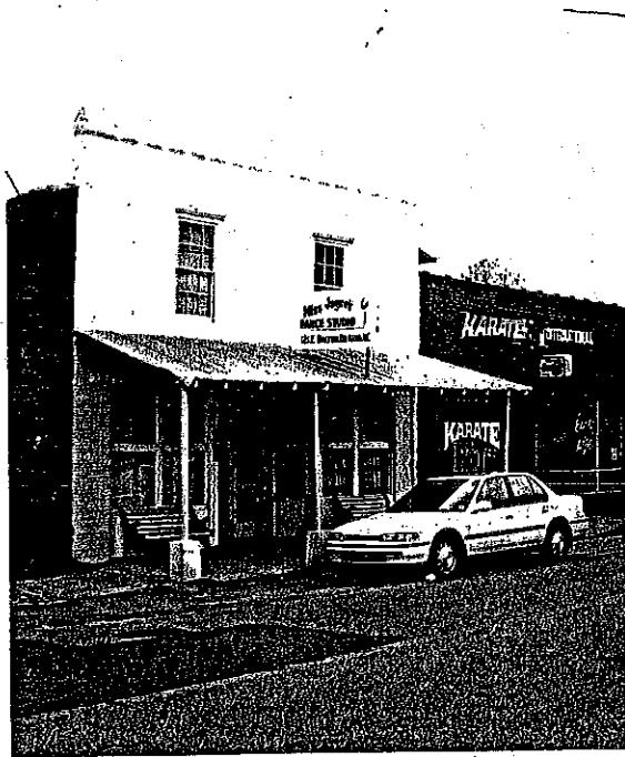
Figure 5. Front wall of 121 East Dalton Road is raised above the roof line, presenting a more imposing urban facade to the street.
