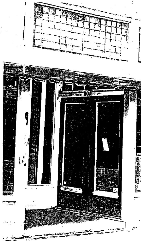
Figure 3. Leaded glass transom at 110 East Dalton Road. Original leaded glass transoms are sometimes concealed behind contemporary signage and can be restored.
