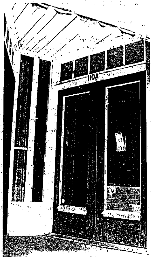
Figure 13. Original wood doors, sidelights, transom, and ceiling at 110A East Dalton Road. The door glazing has interesting wood sills at the bottom. Preserve original wood elements as valuable architectural elements.
