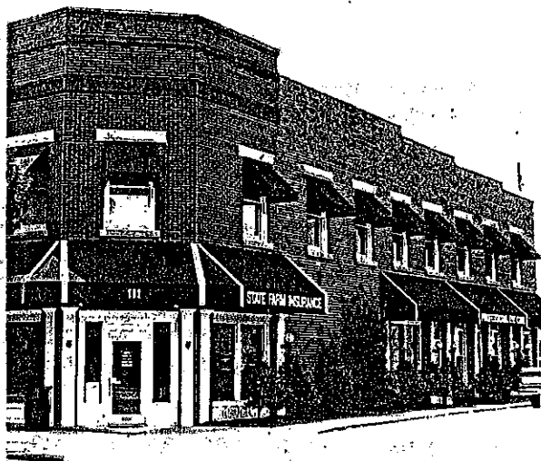
Figure 23. Attractive awnings follow the profile and edges of the openings they cover. Note business identification and street address on awning fringe.
