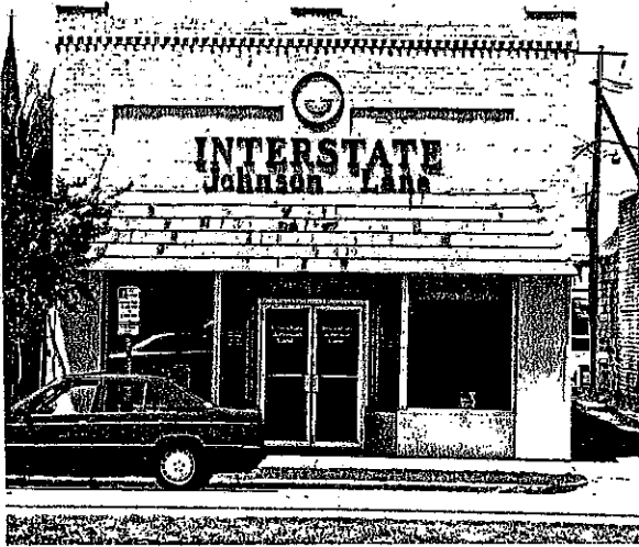
Figure 7. Contemporary cedar shake canopy is an inappropriate addition to this older building. Recessed panels in brick work as sign locations were overlooked. Original storefront glazing, kickplates, and doors have been removed.
